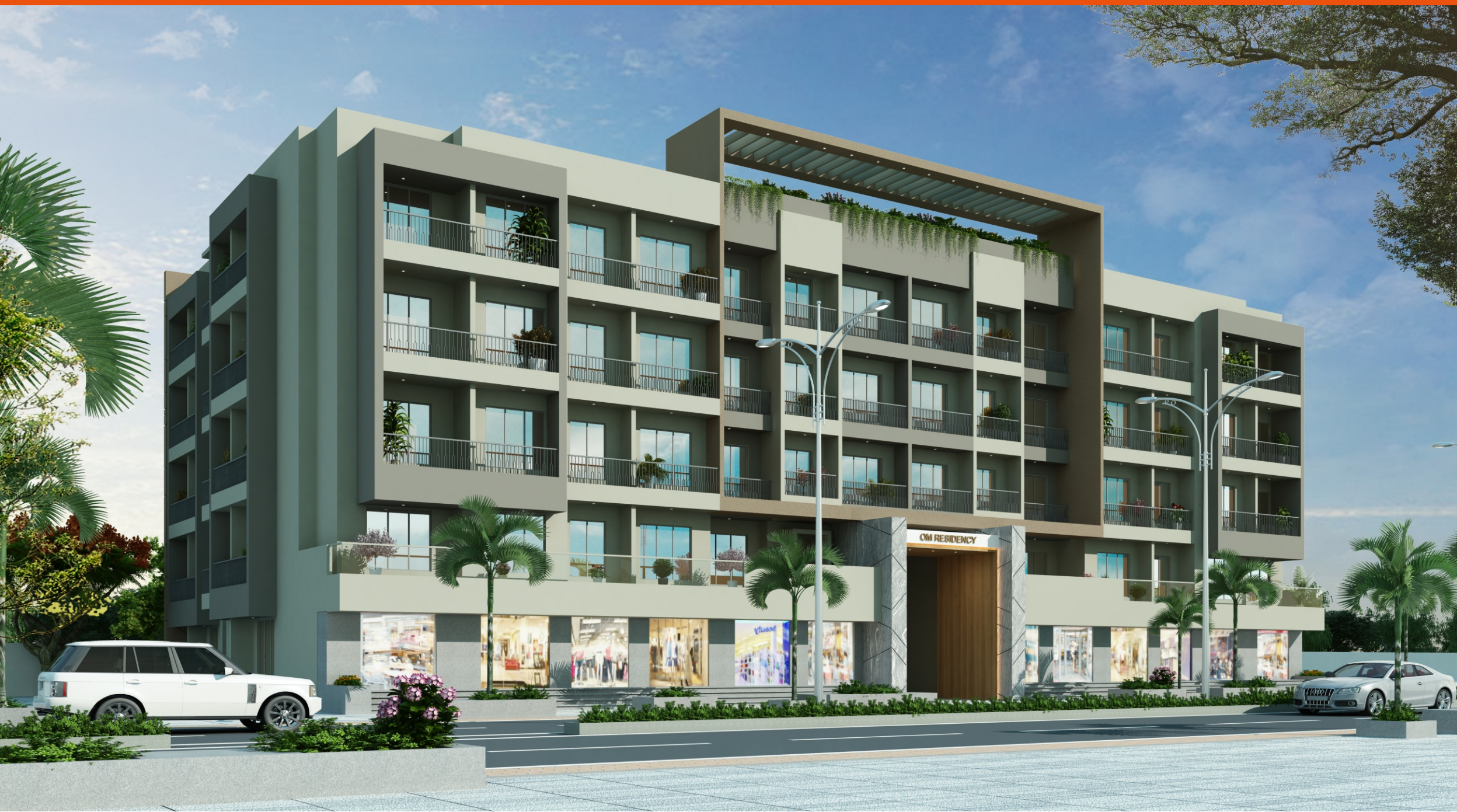
Om Residency Building No. 6
